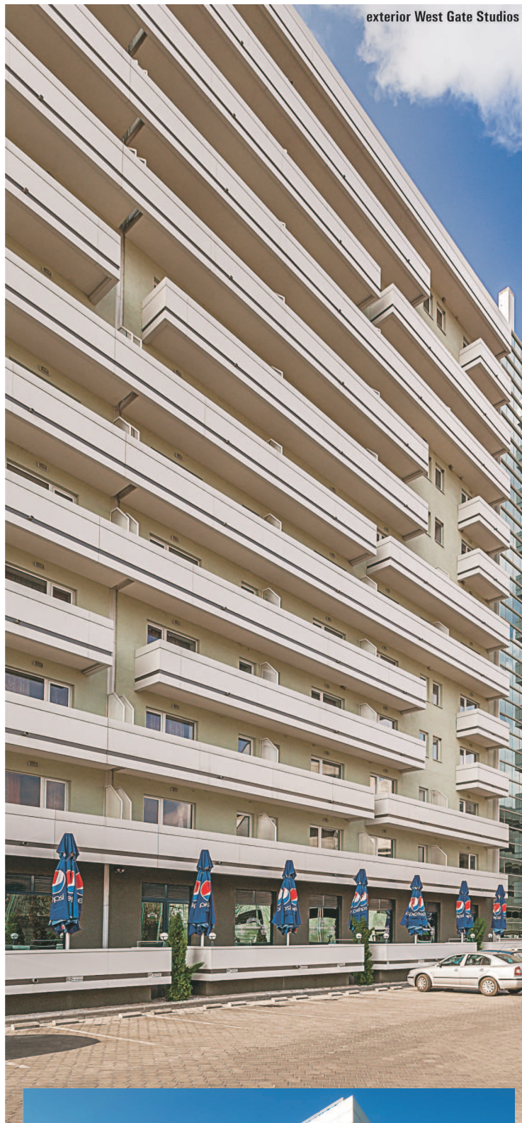
exterior West Gate Studios
